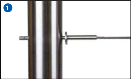
1 Crimp wire into cable tensioner and insert through pre-drilled hole on starter post.
